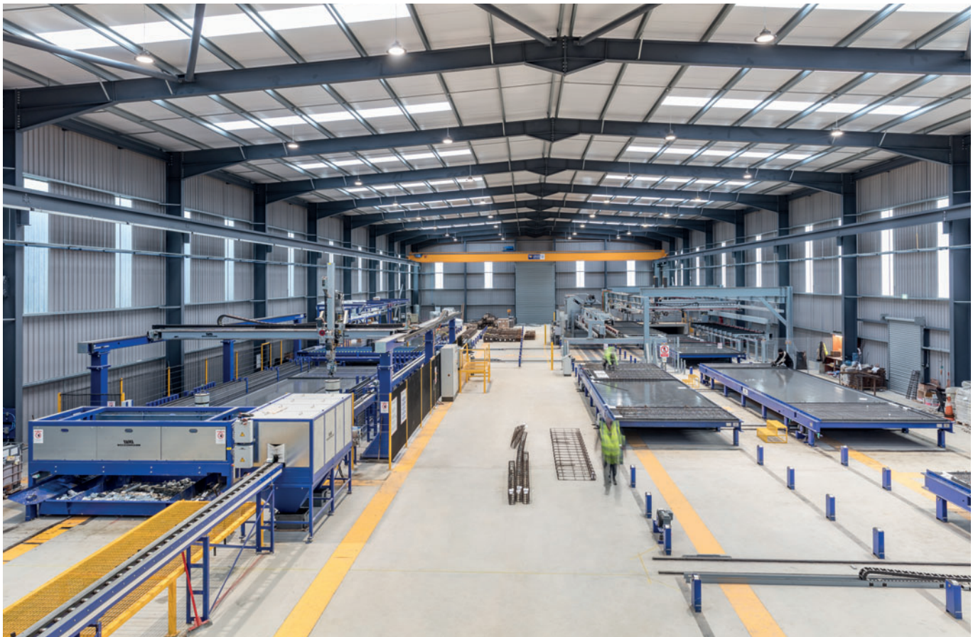
The circulation plant at Keegan Precast in Ireland.
