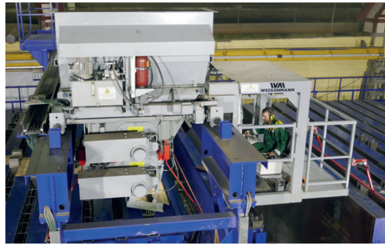
Half-gantry concrete spreader during concreting
