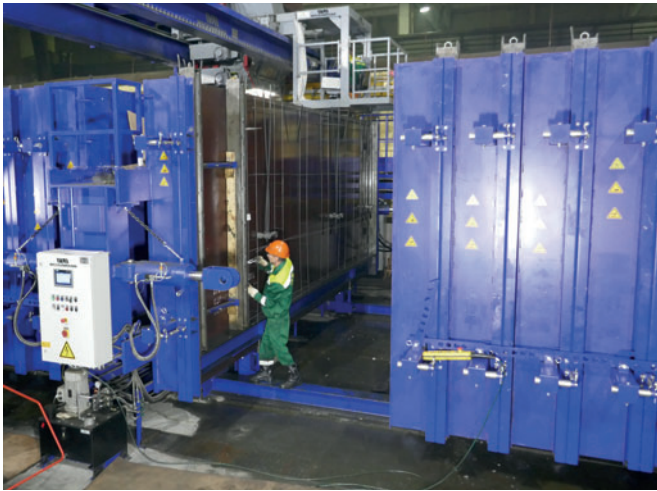
Preparation of the future wall panel
