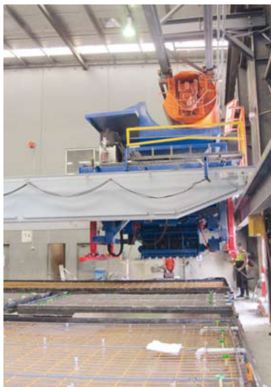
Fig. 1 Concrete distributor taking over the concrete from the bucket conveyor.
